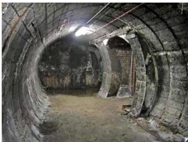
A rare glimpse of the unfinished other side of the lower lift landing. This is not part of the normal public tour. Photo Tim Wellburn
